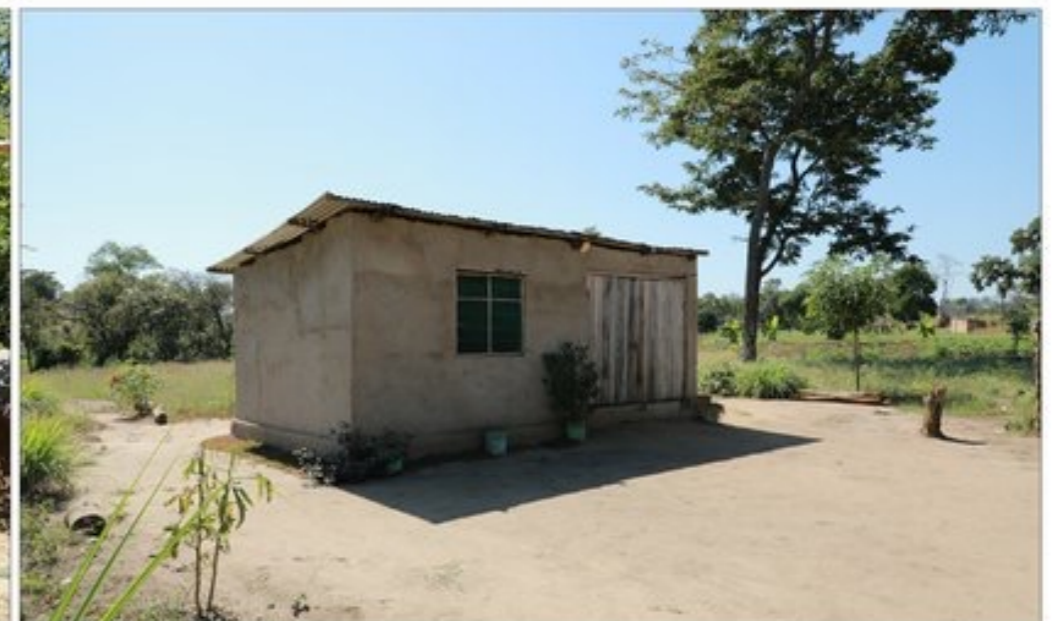
House with metal roofs and plastered brick walls
